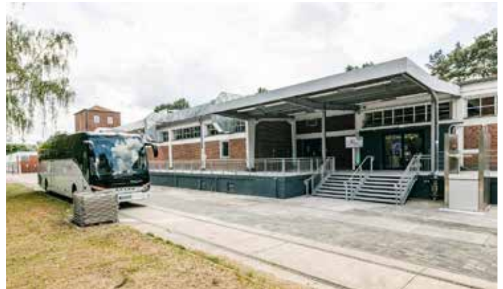
Main entrance (stairs + lift) + outdoor gallery > access to Front Hall
